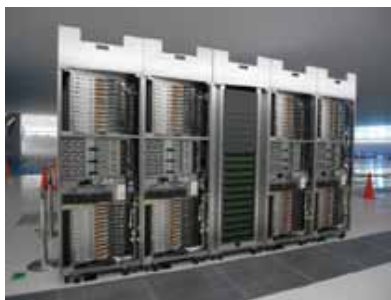
Figure 1. Section of the K computer. Visible are four computer racks with 384 nodes.
